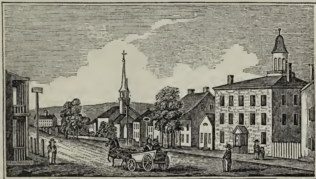
Southeast view in the central part of Schoharie.
